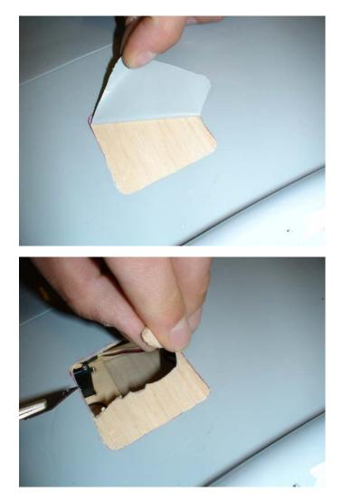
7. Find some off-cuts of balsa or ply which you can use to fit inside the hole, as it will be required to mount the product.
