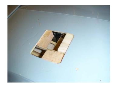
10. Place the frame back in the cut hole in the same orientation as before and draw around the inside also marking all the holes.
